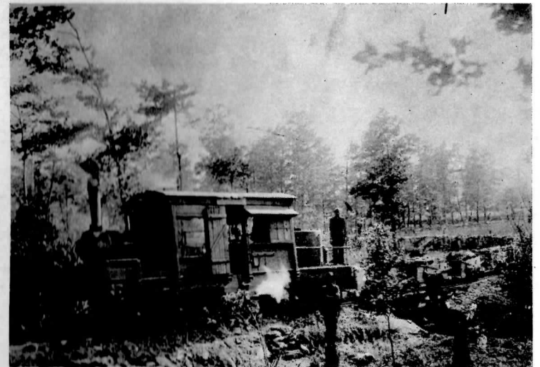
Steam Dinkey used in transporting clay from Mine to Brick Plant
